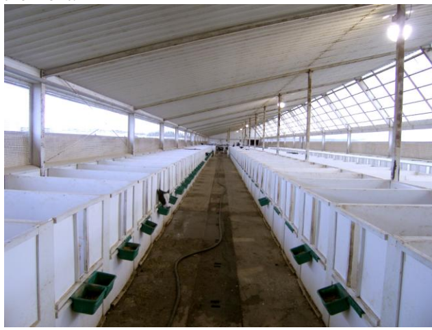
Figure 1. Interior view of a naturally ventilated calf barn with four rows of pens. There is a ridge opening above the translucent-panel roof to the south, adjustable curtain sidewalls, and individual calf pens surrounded by solid panels and a feeding opening in the front.
