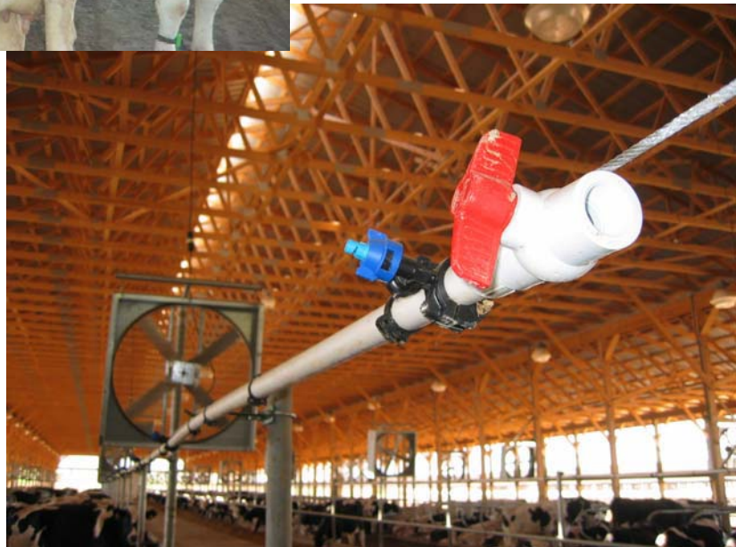
1" PVC with clamp-on style TeeJet Nozzle body with Check-Valve attached to tight ¼" cable
