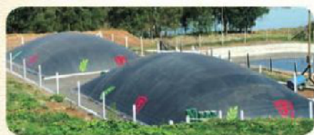
Biogas Digesters - Sao Paulo, Brazil
