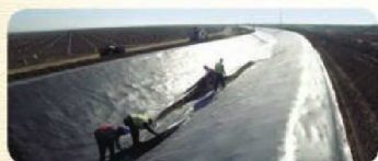
Irrigation Canal - Lost Hills, California
